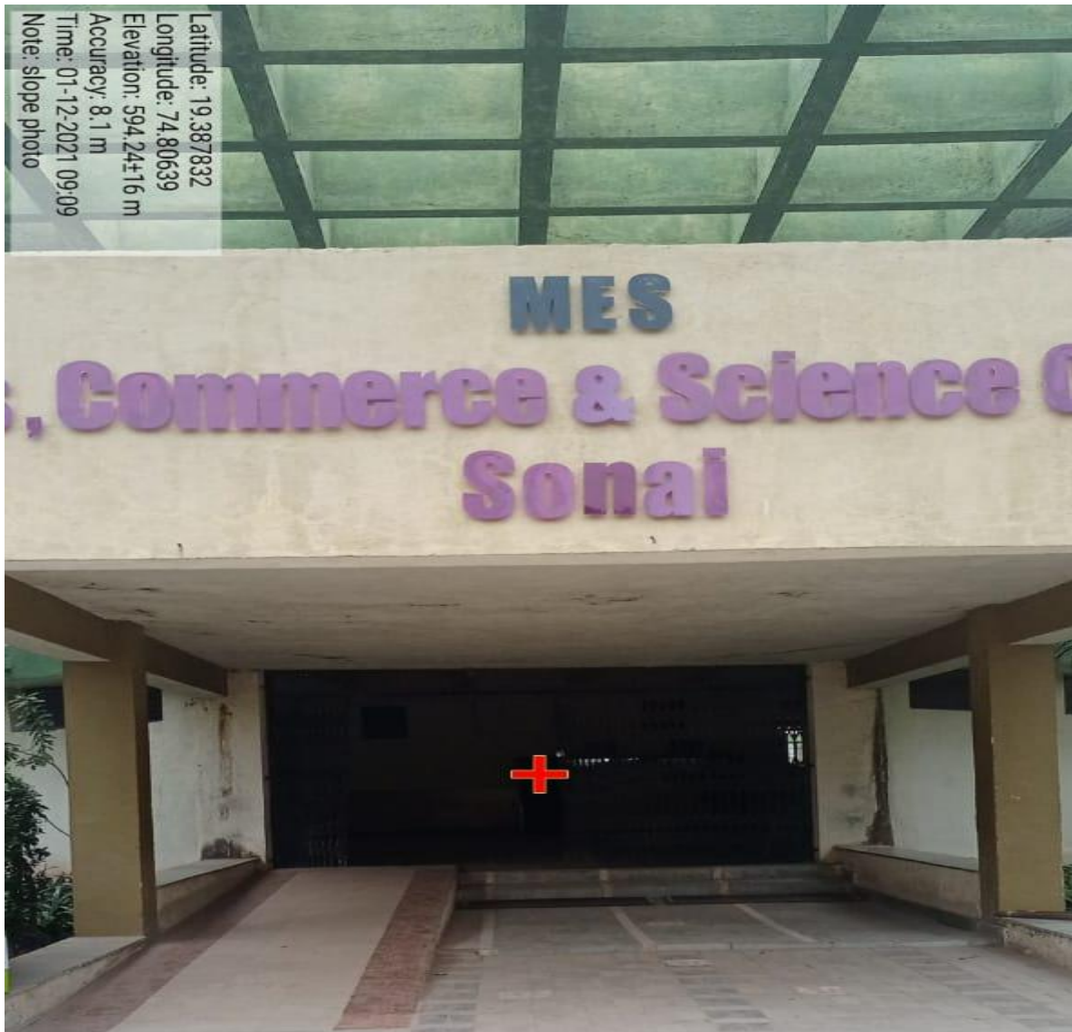
Ramp – Main Entrance
