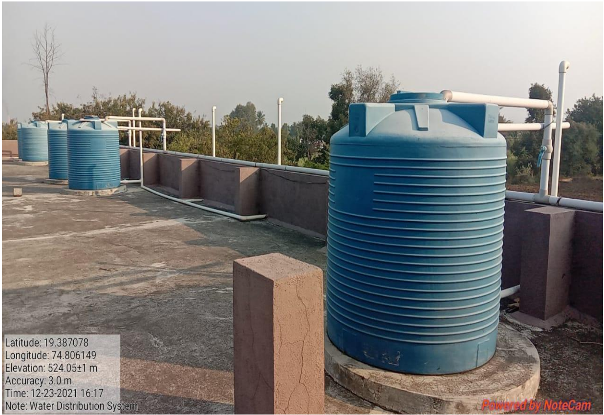
Water distribution system in the campus
