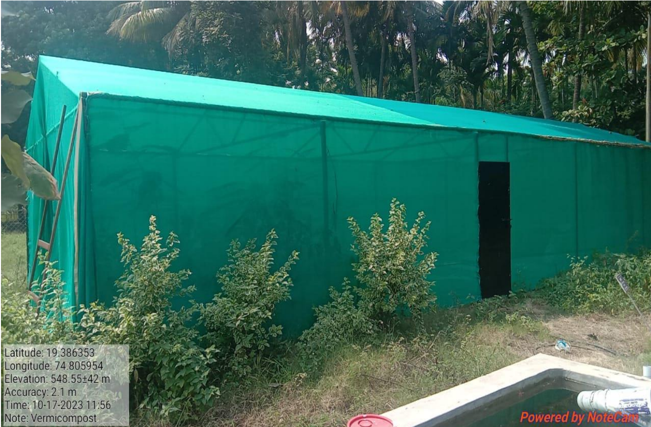
Waste re-cycling system: Vermicompost Plant
