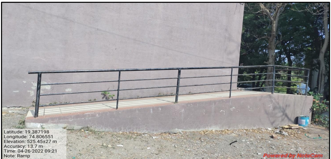
Ramp for handicapped students (Science Building)
