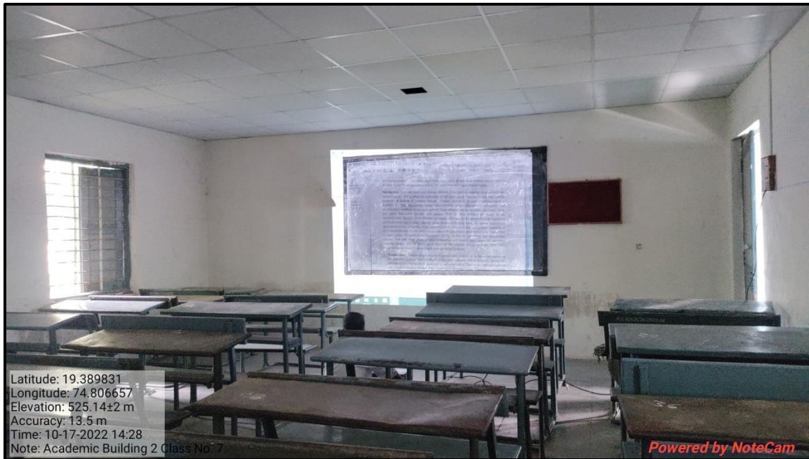
Academic Building 2 Class Room No. 7
